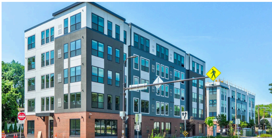
PLYMOUTH AVENUE APARTMENTS MINNEAPOLIS, MN MATRIX DEVELOPMENT, LLC
